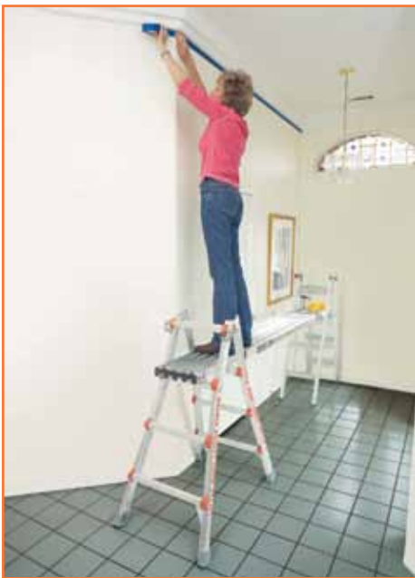
Expand your work area with time-saving scaffolding.
